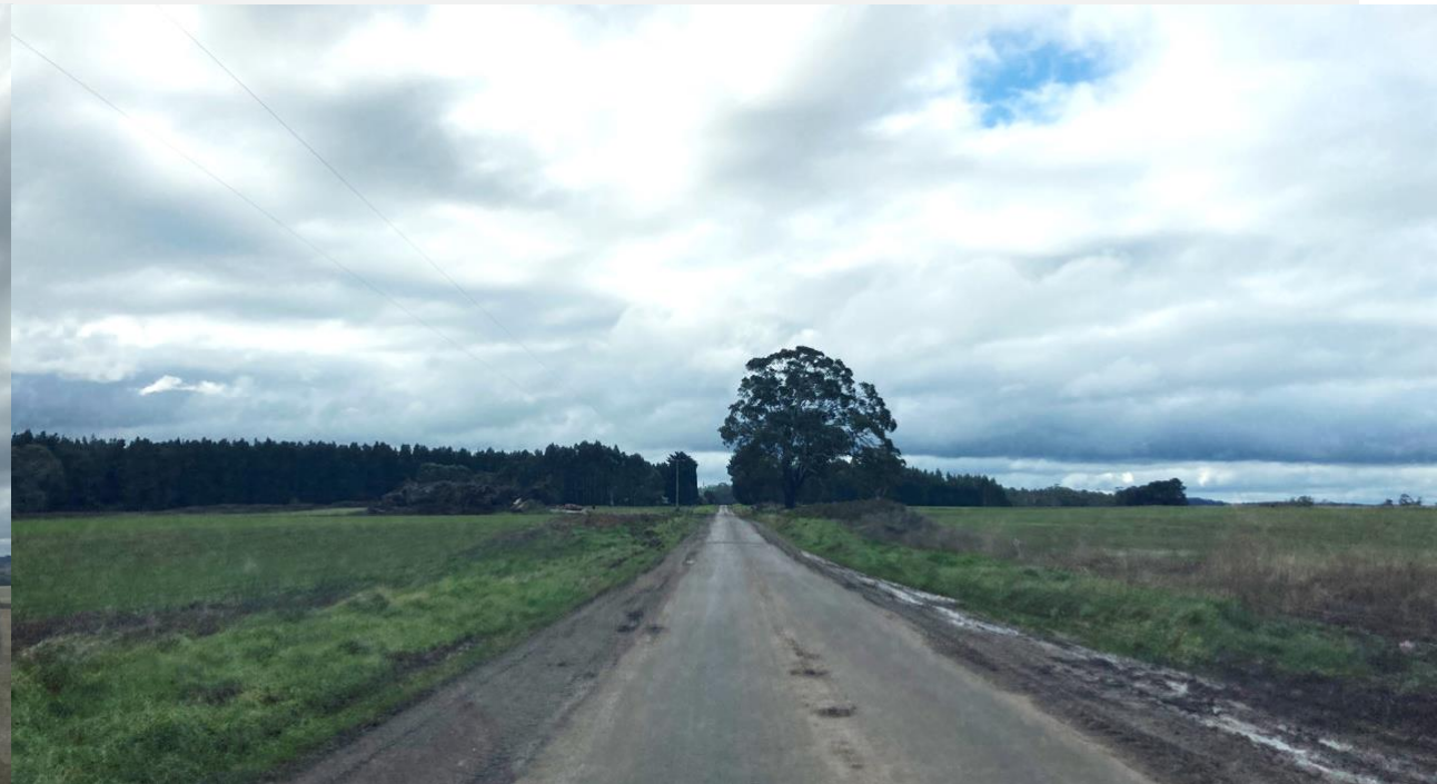
Typical example of a narrow pavement/sealed road within the study area
